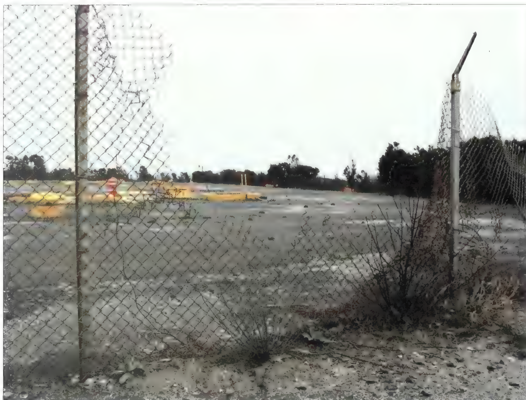
Figure 5.122. View looking northeast across missile magazines, NIKE launch site. After vegetation removals the inner, outer, and kennel fences should be inspected, repaired where needed, and replaced where damaged or severely deteriorated (Olmsted Center, April 2008).
